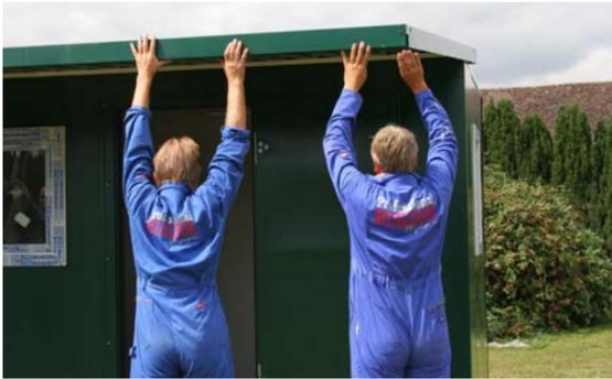
c. Lift the roof onto the cabin and manoeuvre until it clicks into position.
