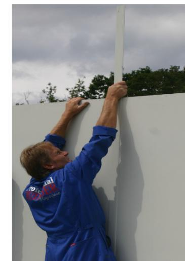
f. Then insert 'H' Section joining strip, insert at the top of 2 joining panels...
