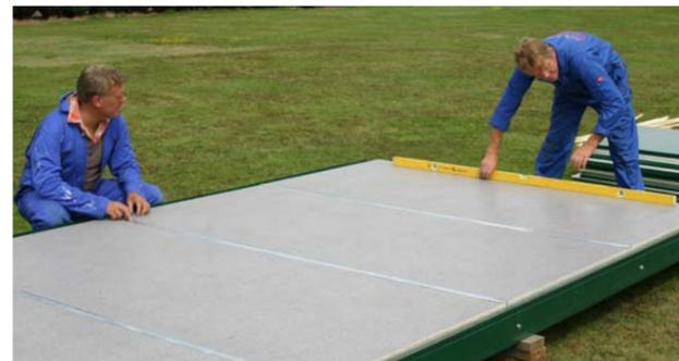
f. Site the chasis where you want to assemble the Cabin, check that the floor is level with a spirit-level, this is crucial for the smooth assembly of the unit.
