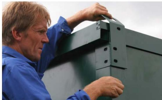
d. Fit the lifting eyes to each corner to hold the roof in situ.
