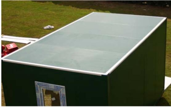
a. The roof is now ready to have the roof cap fitted.
