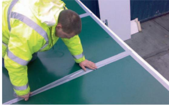
b. Seal all joints of the roof with the silver tape.
