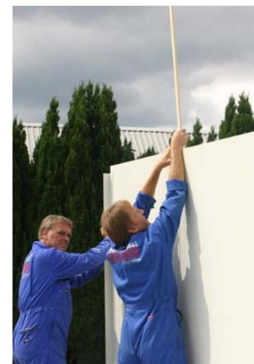
e. Insert a single wooden batten between each wall panel.
