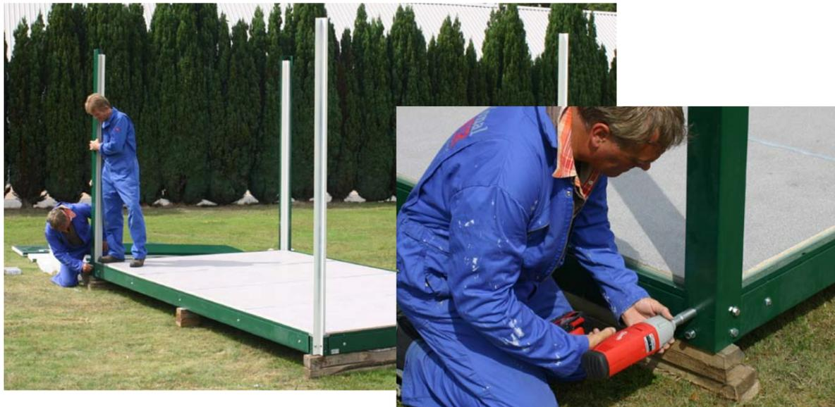
c. Screw in, but don't tighten completely, yet.
