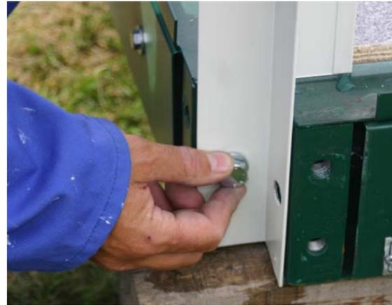
b. Align and fit the 4 corner outerposts, using the self tapping bolts, 4 for each corner.
