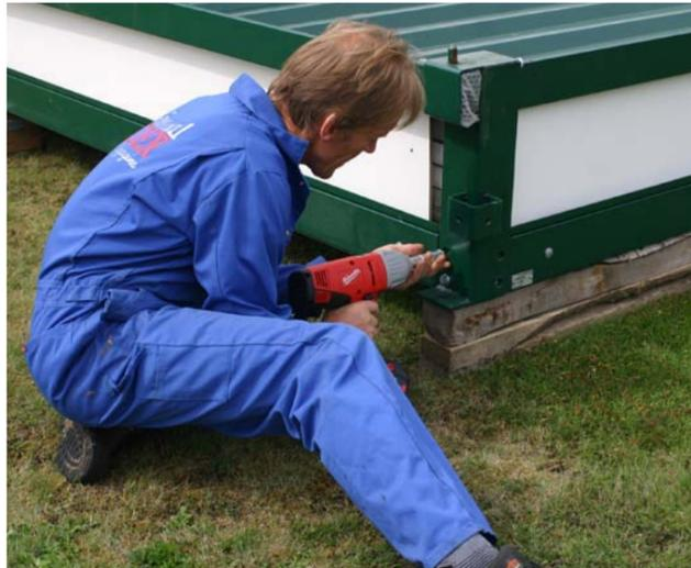
c. Remove the top panel (roof).
