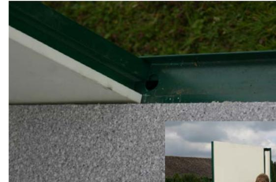
d. Line up the wall panels into the groove and slide into position, repeat this with the remaining wall panels.
